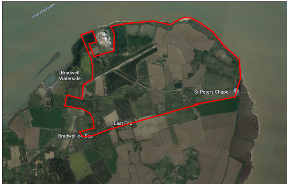
Fig 1: Approximate Location of Bradwell B Nuclear Power Station Site.
